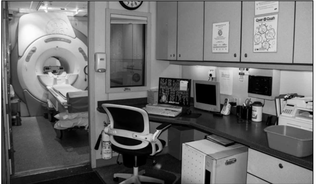
The mobile magnetic resonance imaging (MRI) unit that visits the Health Center contains an MRI scanner and separated office space from which staff operate and monitor the scanner.
