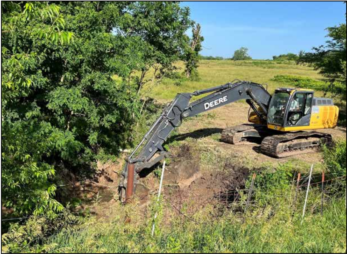
The photos above show heavy machinery being used under the bridge over N Road to reduce erosion and to smooth out the area making it safe for buffalo to cross the stream under the bridge. This allows the animals to move between pastures for rotational grazing.
