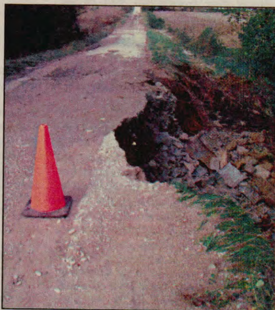
This photo shows how part of the roadway was actually washed out from the rains. This photo was taken on O Rd just off of 134 Rd facing north.
