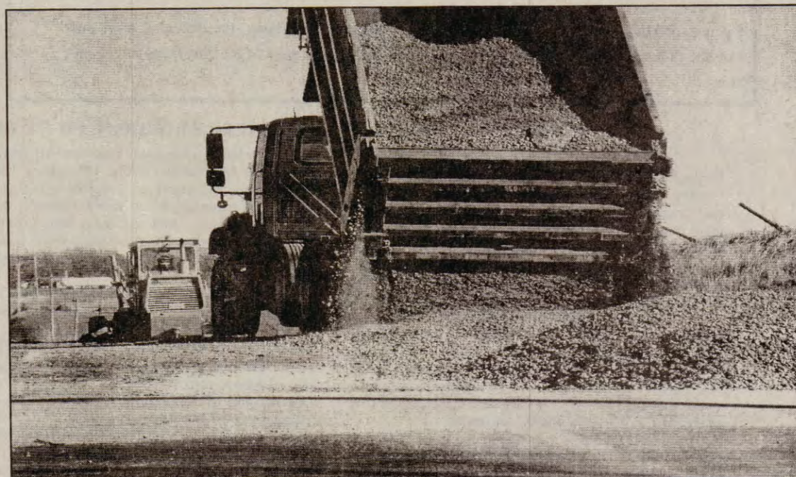
Major work has been done on 162 Road and Q Road by the Road and Bridge crew. Wear and tear plus the recent rains have left the dirt road in need of rock. The photo shows the dumping of rock with the grader used to level out the rock.
