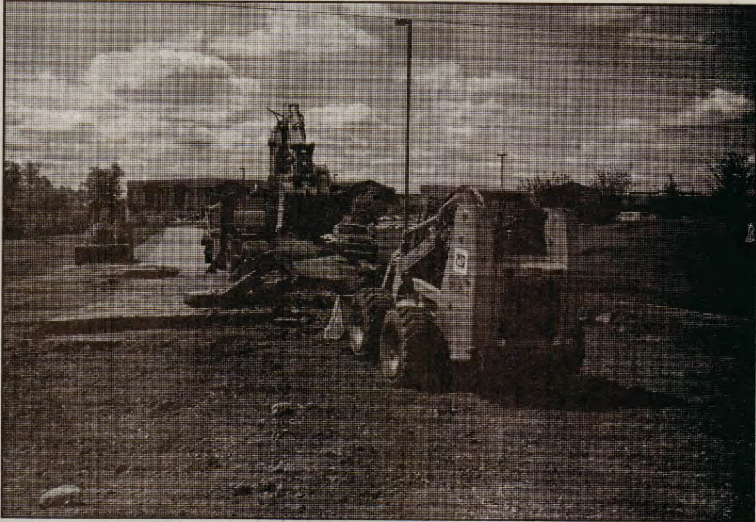
The Road & Bridge Department recently fixed a water drainage problem that was causing the casino's entry road to buckle and was also damaging the surrounding landscape. The work consisted of tearing out a portion of the road, installing crossroads tubes and then reasphalting the road. The work caused the entry road to be closed for a short time on May 9 but it was reopened the next day.
