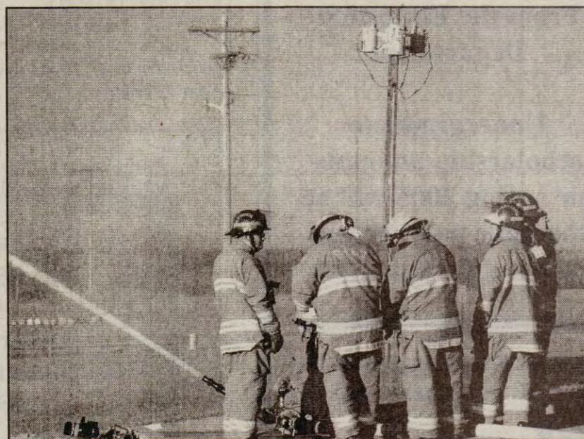
PBPB Emergency Service Dept. crew training with the Ground Water Monitor (GWM). The crew is able to continue fighting the fire without having to go directly into a dangerous situation with the GWM; it is placed near the fire with a couple of hundred feet of hose that is connected to the engine. An unsafe scene would be anything in a closed container such as Hazmat, propane and oxygen bottles.
