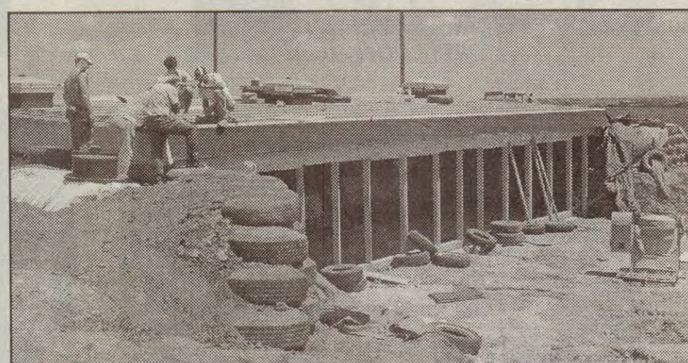
The Earthship building is located on 142nd Road near the Solid Waste Plant and is proposed for use as a water quality laboratory. Note the old tires (left) that comprise a large part of the structure. In the photo above are some other Civitas members who were helping Wold on the day that this photo was taken. The PBPB Maintenance and Construction Department and several other departments also helped build the structure.
